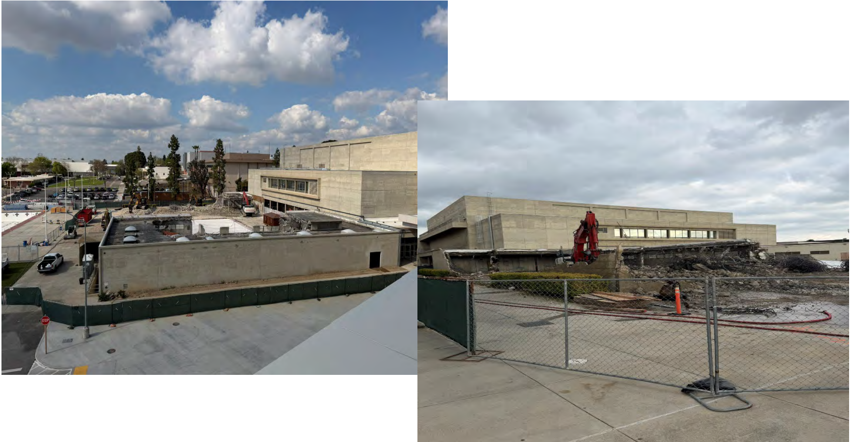
Combined Gym and Field House Pool Equipment Building Construction Completion March 2027
