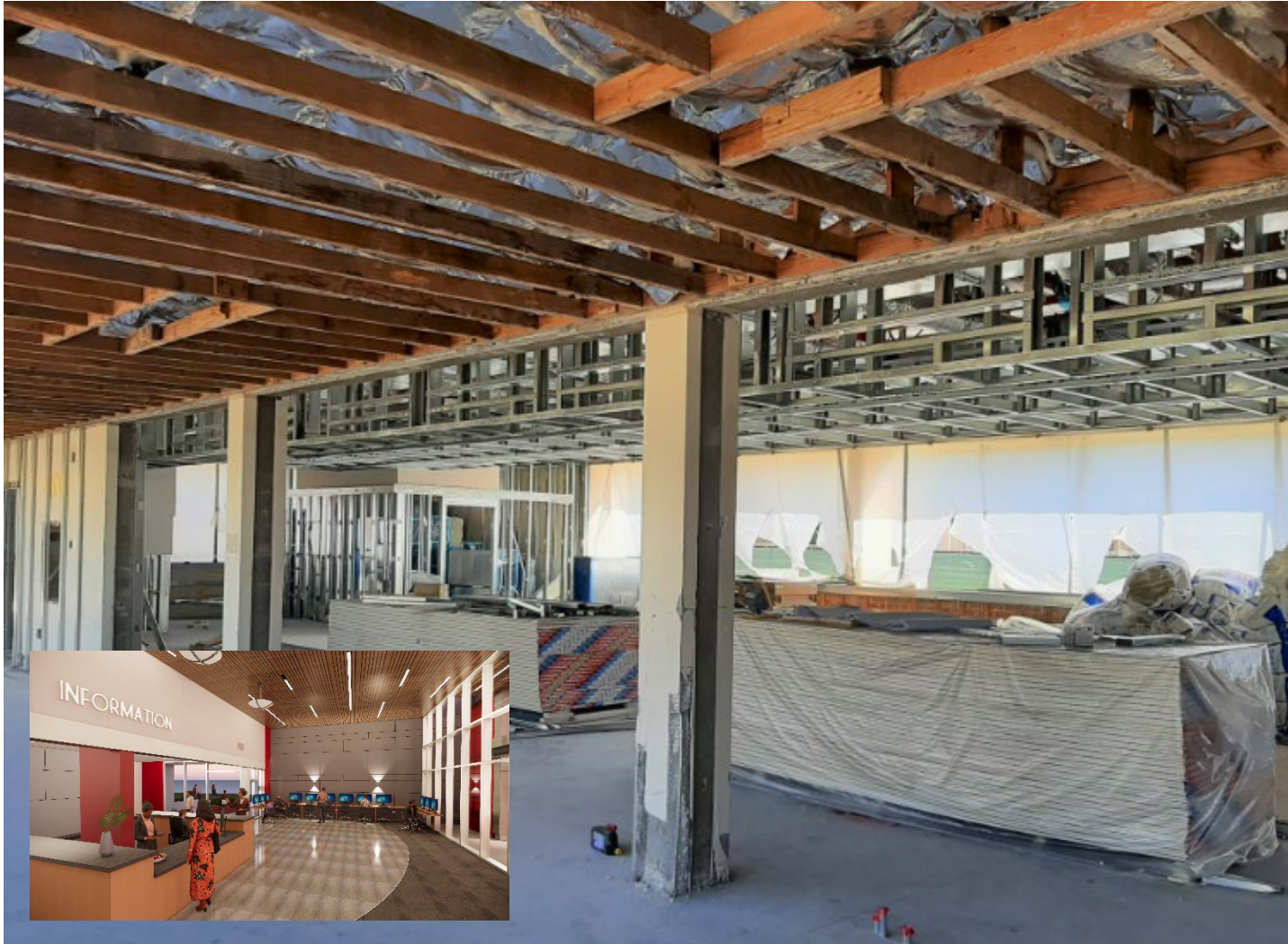
Welcome Center - Construction Complete November 2023
